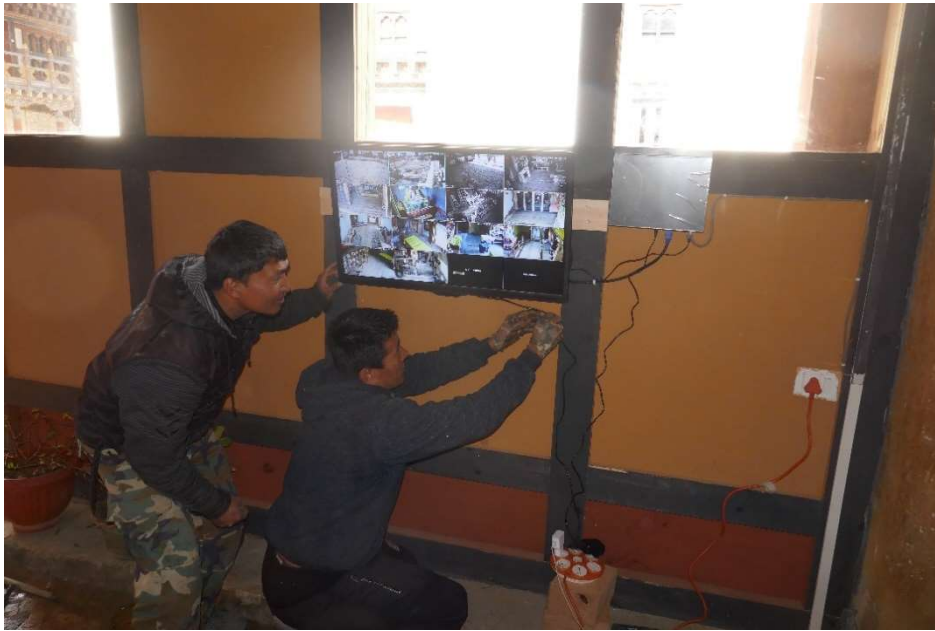
Installing CCTV system
